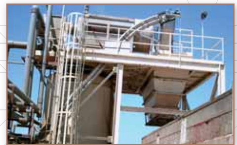
Double bend - tomato waste conveyor.
